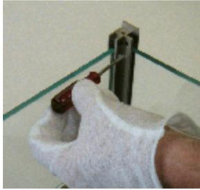
Tighten the white nylon setscrews that secure the rear glass and side glasses. Turn clockwise to tighten.
